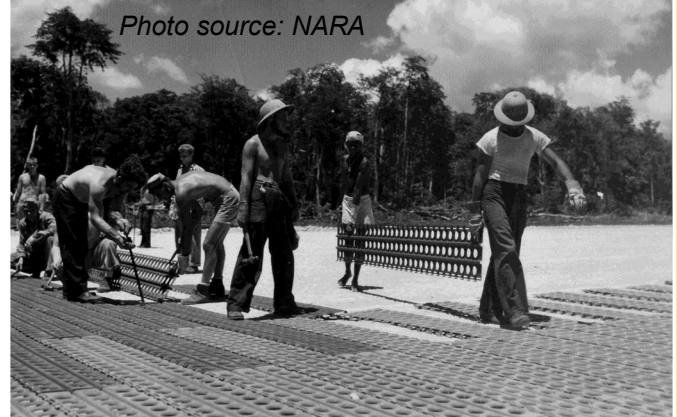
Image: Marston Mats being laid by Seabees and Ni-Vanuatu workers on Bomber 02 (Peko Airport) 1943
