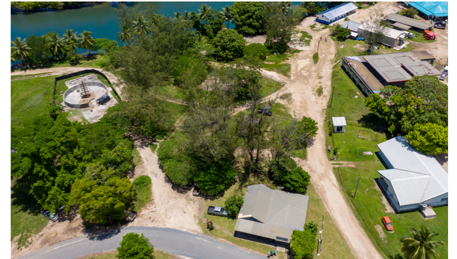
The Museum site beside the Sarakata River. The current Mini Museum is in the building towards the centre, at the bottom of the photo.
